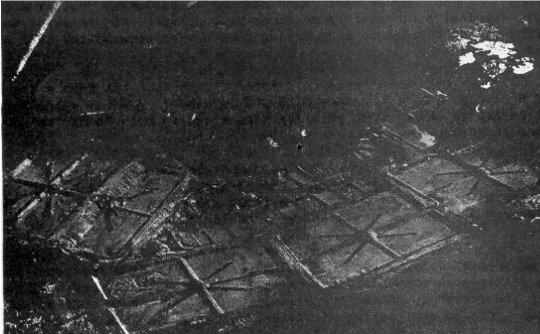
Figure 2-17. Aerial view of wastewater treatment plant with intermittent sand filters. (In each set of four beds, distribution troughs for dosing radiate from a central diversion box.)
