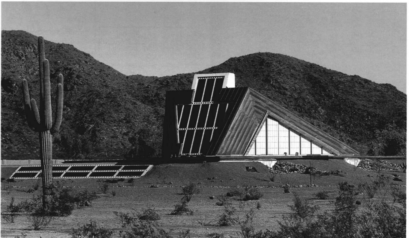
A house with a solar panel heating system.
